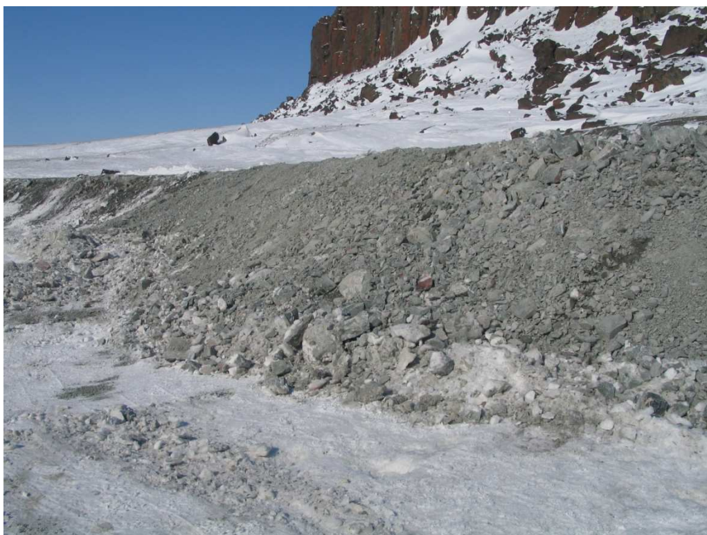
Photo 5: Location of ramp after backsloping
