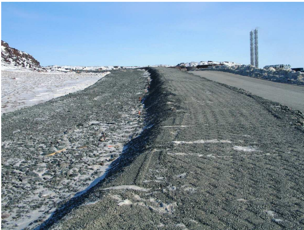
Photo 2: Berm, finished product. Crush on surface has been packed. Sta 0+15 facing east.
