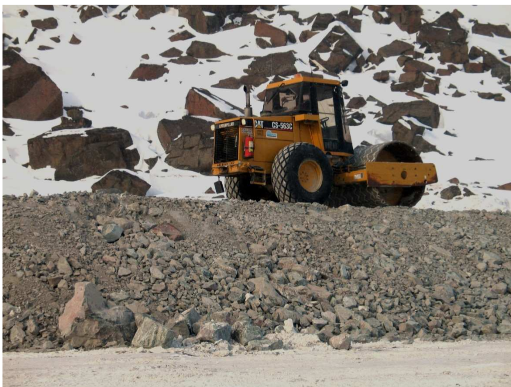
Photo 7: Packer working ~ Sta 5+00
