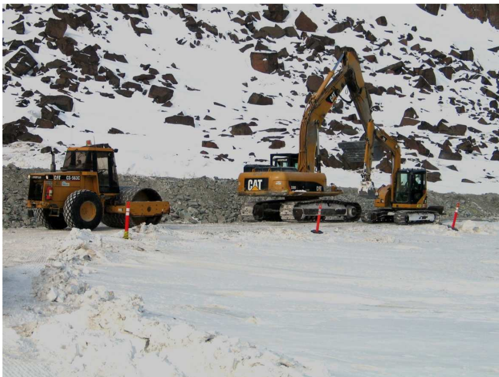
Photo 6: Constructing ramp to permit packer to get up on berm.
